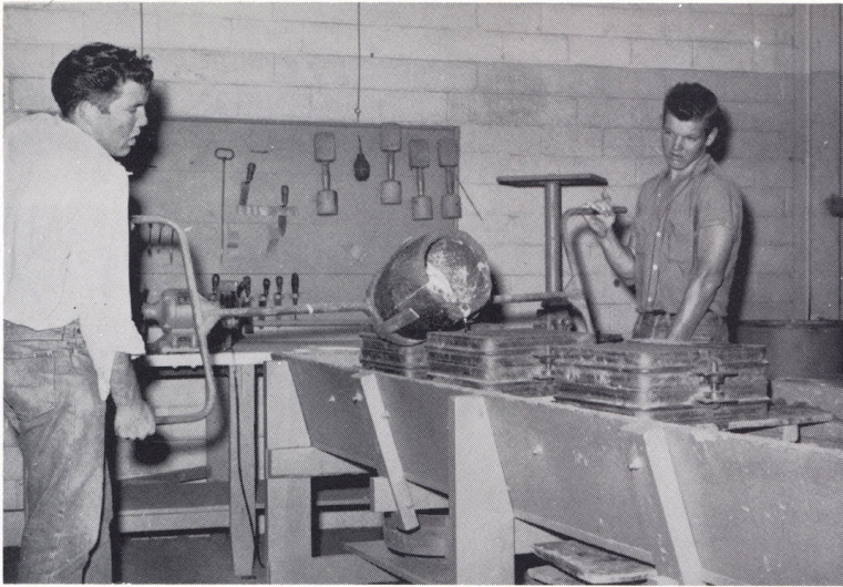
Oran Bunch and Bobby Nelson are shown pouring metal.
